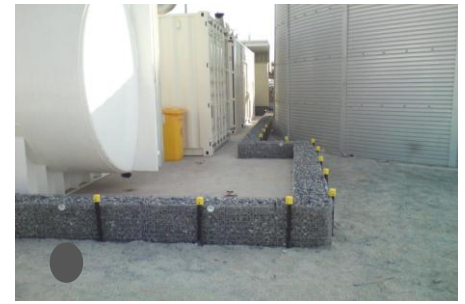
Gabion Bund Wall
