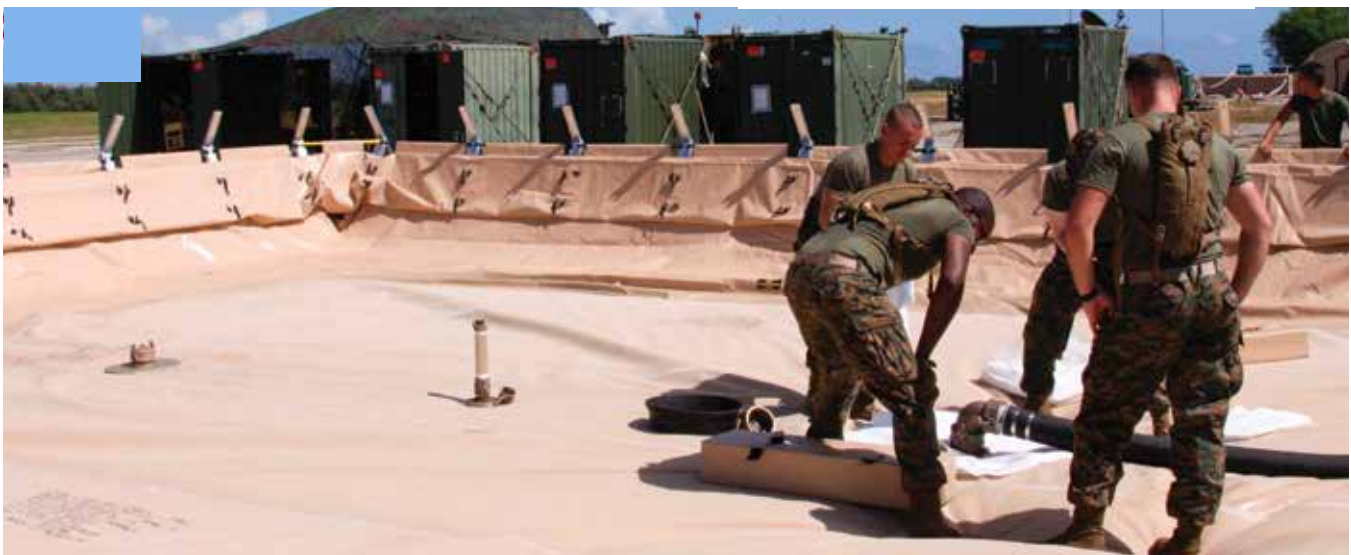
Fuel being transferred from a tanker to a storage bag with the All Terrain Berm™ providing secondary containment.
