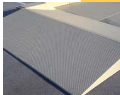
Integrated exterior ramp.
