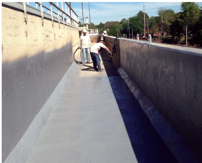
Spray-on technology coats smoothly to repair cracks and leaks—tack-free in seconds
