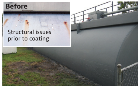
UV and corrosion resistant high-strength coating for tanks
