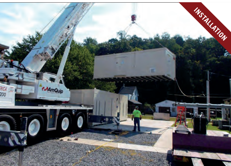
Modular chemical storage building with double leaf doors, mechanical ventilation, and integral dry chemical fire suppression systems.
