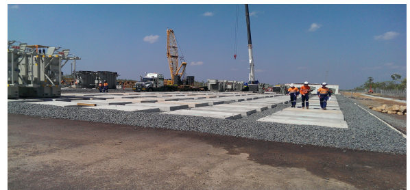
Large above ground storage site applications
