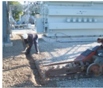
Dike installation for oil and rainfall requirements.
