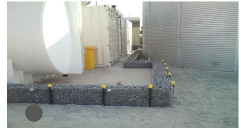
Gabion Bund Wall
